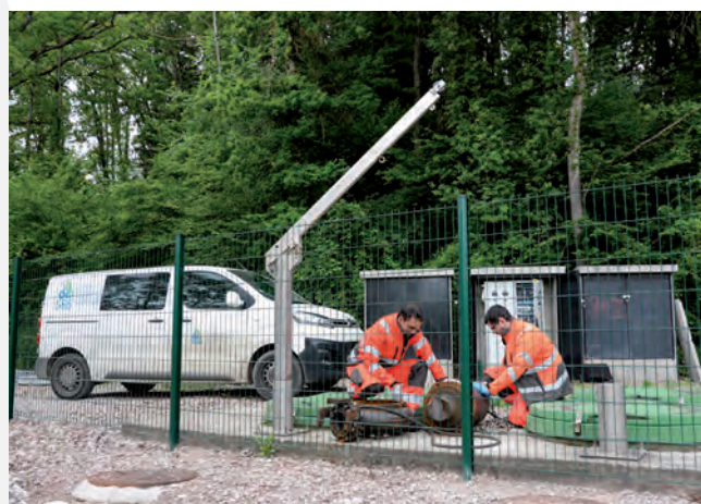
Intervention pompe relevage
